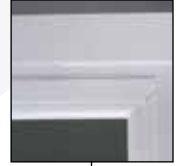
Fusion-welded Panel Construction
