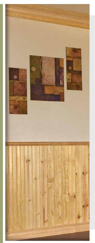
Finger-Joint (FJ) Pine consists of small pieces of wood that are recycled and jointed together to create lengths for door casings and 16' or 17' lengths for crowns, base and chair rails. This allows for ease of installation and less installation joints, typical of solid woods.
